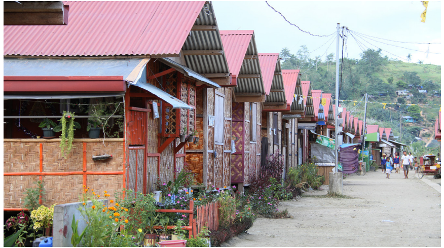
Two years after Super Typhoon Haiyan slammed into the Philippines, claiming 6,201 lives and leaving entire swaths of Leyte and Samar islands in ruins, CRS had repaired or reconstructed 20,000 homes. Photo by Kim Pozniak/CRS
